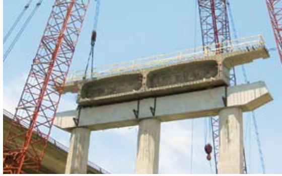
End segments for the main spans were precast on the footing below their final location and lifted into position. Photo: Traylor Bros.
